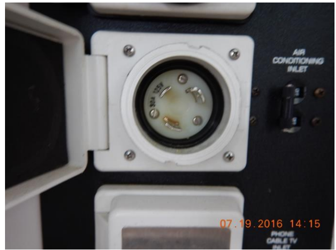
Figure 28 - Air Cond Shore Power Inlet connector excessive heat damage
