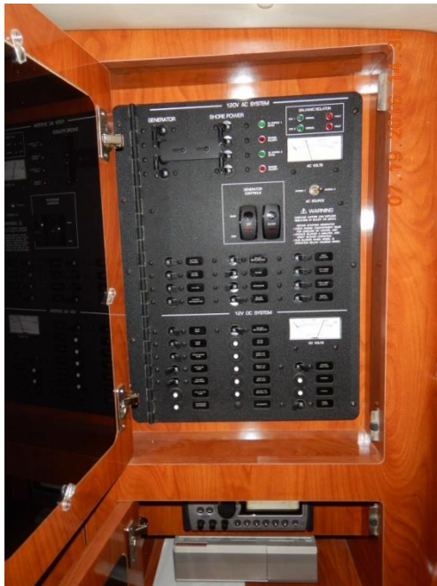
Figure 29 - Main Electrical Panel
